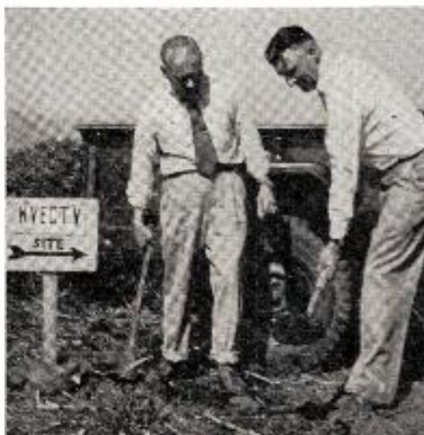
WITH PICK and shovel, KVEC-TV San Luis Obispo, Calif.'s Station Manager Les Hacker (l) and Commercial Manager Jack Wasson break ground March 18 for the new station's site, located north of the city. Tentative date for programming to start is May 8, which is the 16th anniversary of KVEC-AM.
